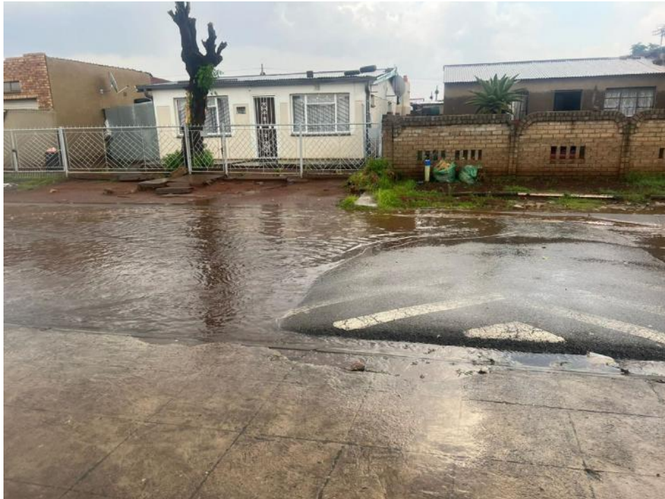
Figure 1: Flash flooding in a Katlehong street due to poor drainage
